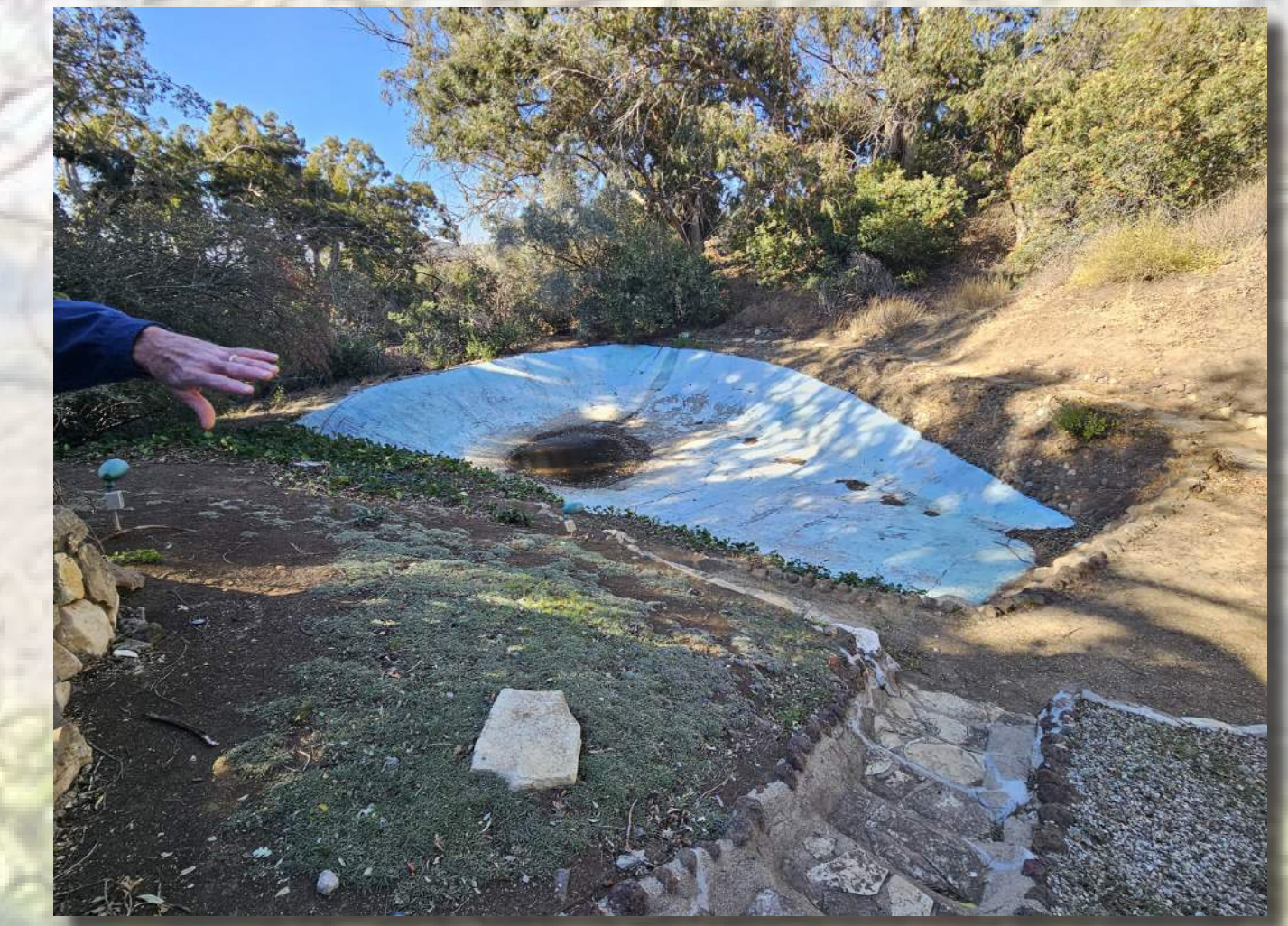
REPAIR/RESTORE POOL (2026 Est. Cost $20,000)
