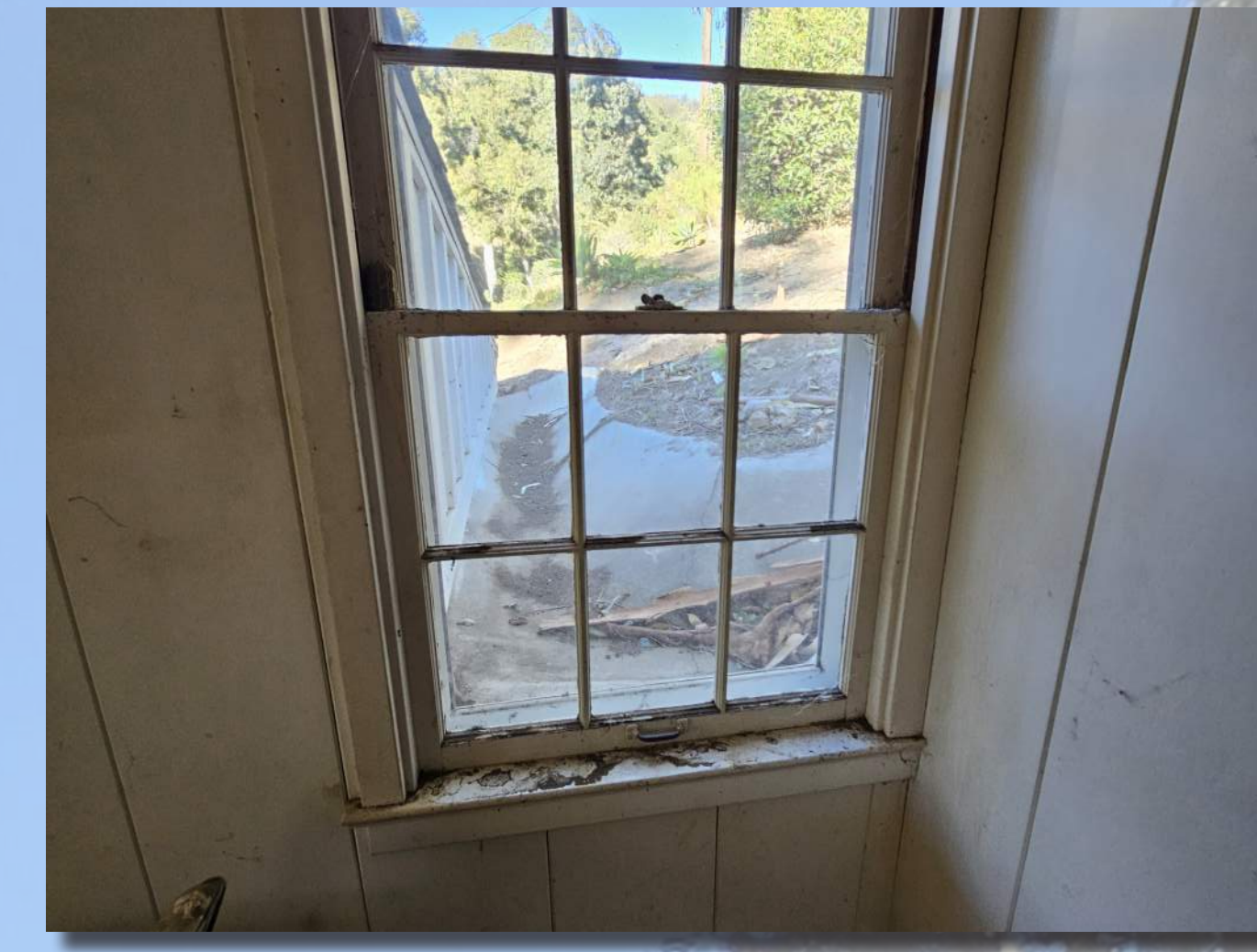
REPAIR/RESTORE WINDOWS AND DOORS (2026 Est. Cost $59,000)
