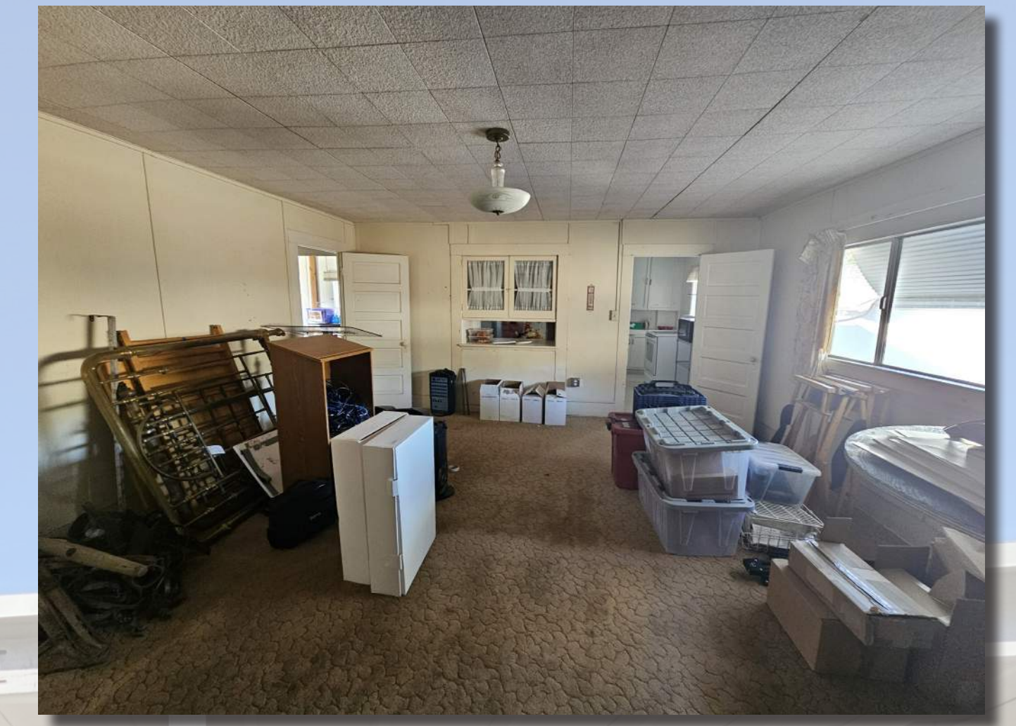
REPAIR/RESTORE FLOORING (2026 Est. Cost $5,000)
