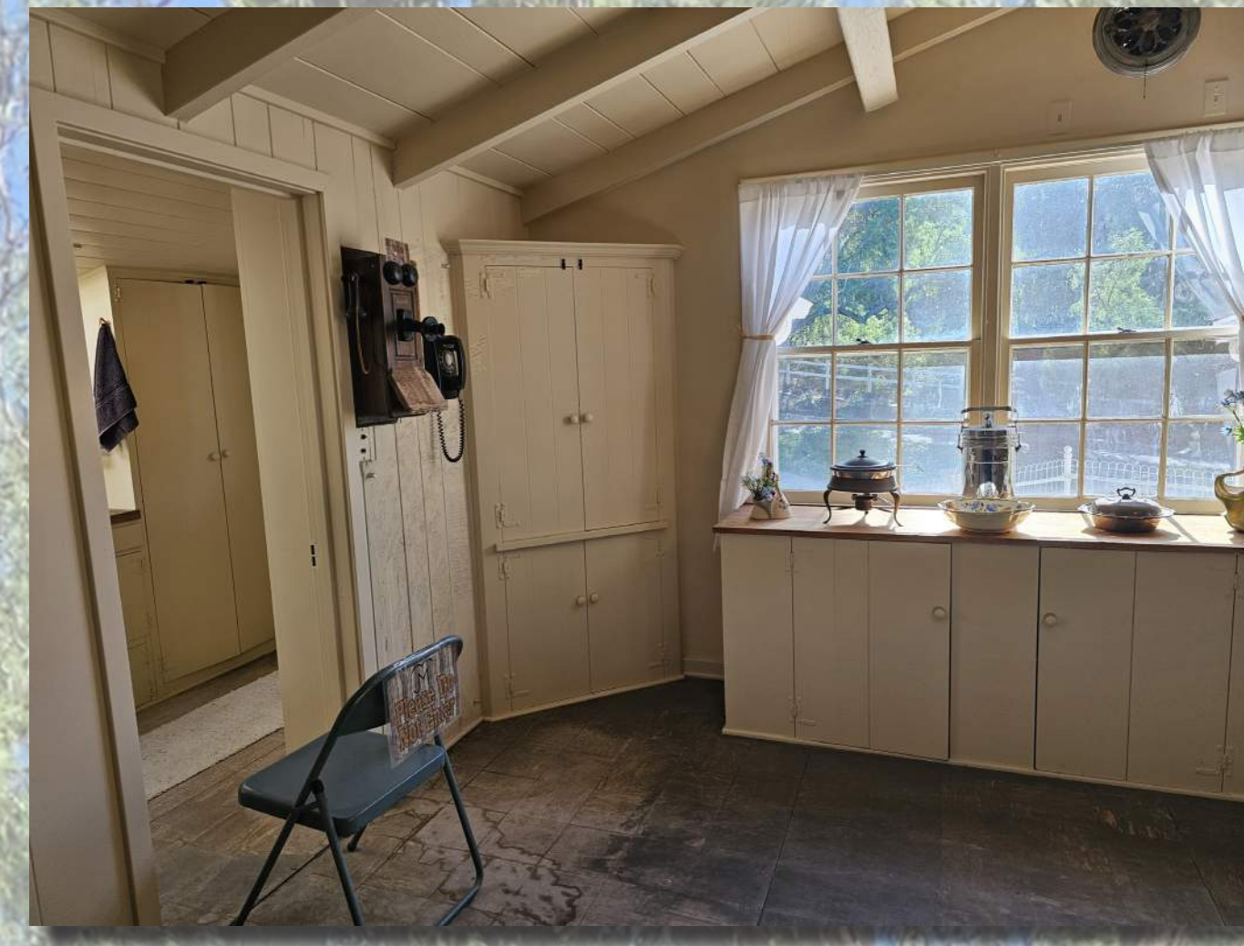
REPAIR/RESTORE FLOORING WITH PERIOD-SPECIFIC FLOORING (2026 Est. Cost $23,000)
